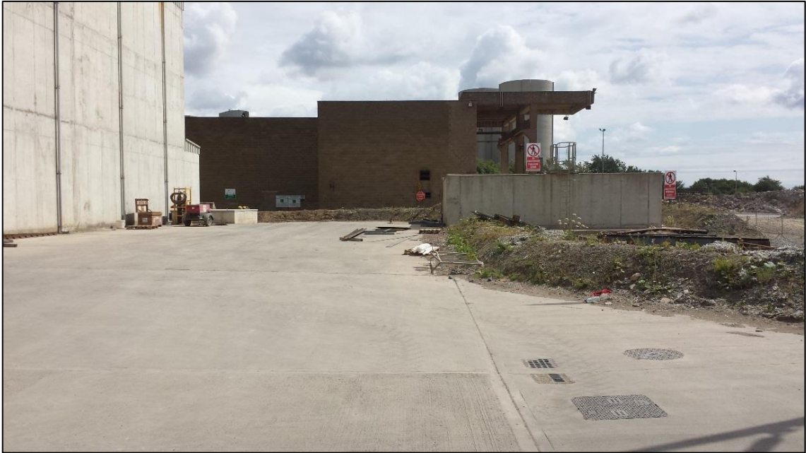
Photo 11.4: View of Area 3 looking west.
