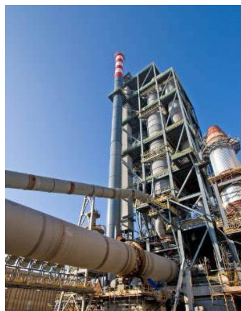
Plate 3.2 Photo of Preheater tower and Kiln 3 at Platin
