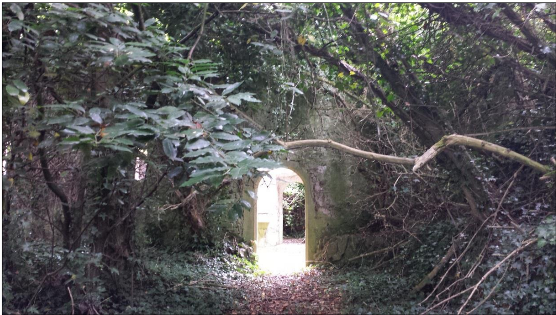
Photo 11.1 View of the entrance to Platin Church ME027-003001 - facing south
