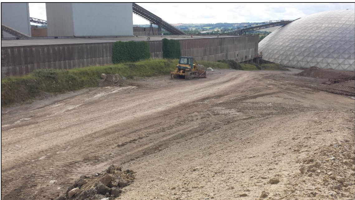
Photo 11.3: View of Area 2 looking south-east.
